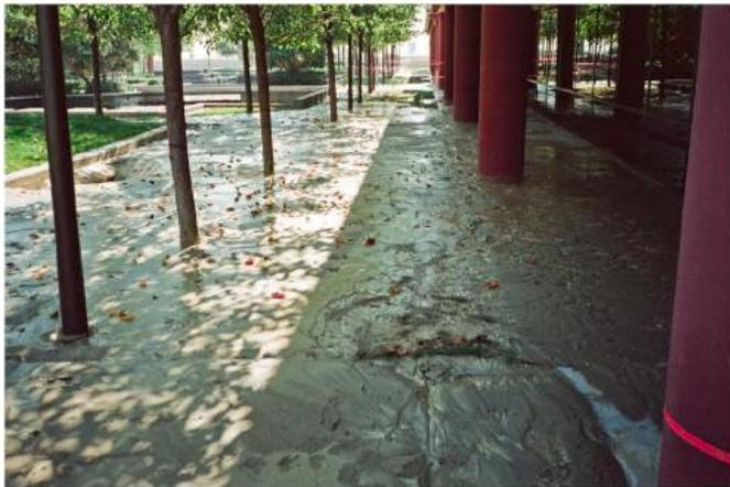
Fig. 24. Example of liquefied sand transported to the surface of the building periphery (1320 Harbor Bay Parkway).
