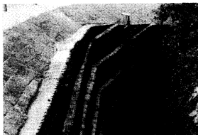
Photo 5. Stretch-made polymer grid (SR) reinforced embankment in Japan (the foremost one in 1985)
