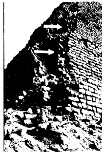
Fig. 11 In the corners, remains of buttress walls
